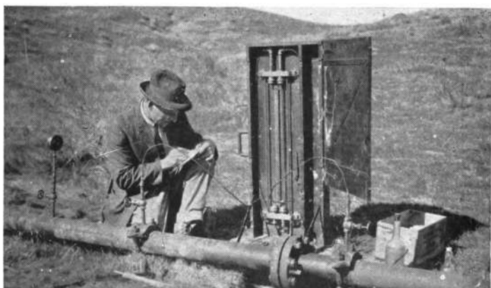
Fig. 49—ORIFICE FLANGE METER AND LIGHT PORTABLE DIFFERENTIAL GAUGE, PIPE TAP CONNECTIONS
