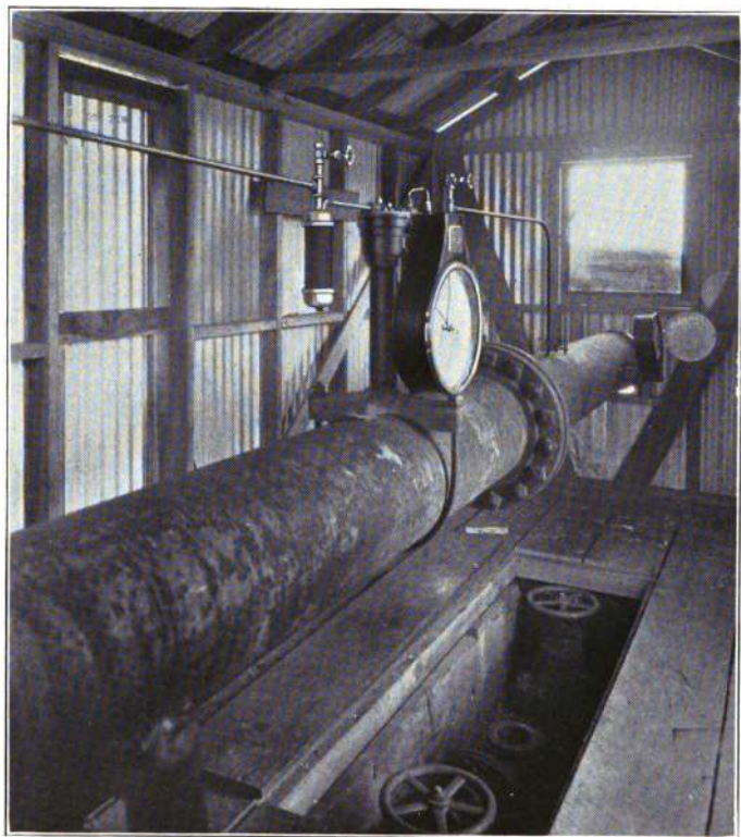
Fig. 11—ORIFICE METER ON LARGE GAS MAIN
