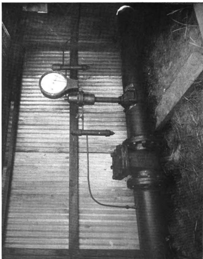
Fig. 96—ONE OF THE FIRST INSTALLATIONS OF ORIFICE METER BODY AND 60 INCH DIFFERENTIAL GAUGE 2\frac{1}{2} and 3 Diameter Connections
