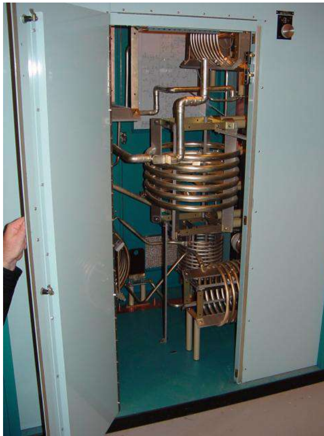
Figure 3.18: High power inductors formed from hollow tubes.
