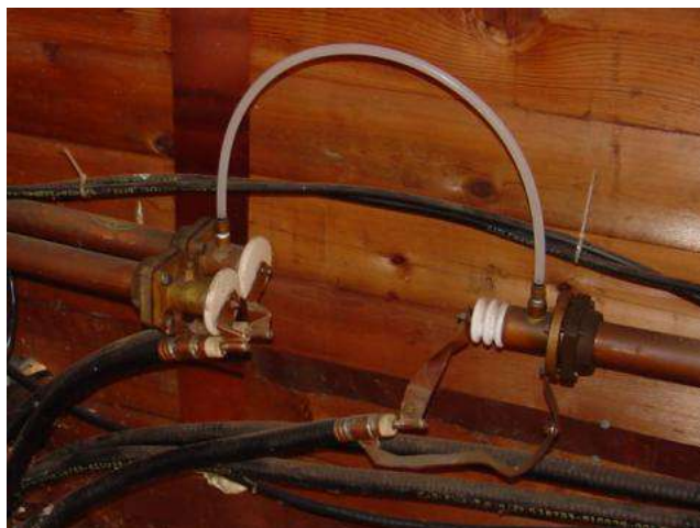
Figure 14.52: Flexible coaxial cables connected to rigid lines.
