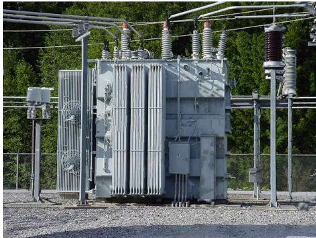
Figure 9.20: Substation transformer.
